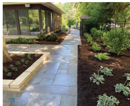
New paved walkways
